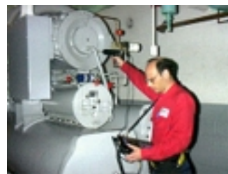
From steam trap faults and valve leakage to compressor problems, ultrasonic detection can be used to find a variety of problems that generate ultrasonic signatures.
